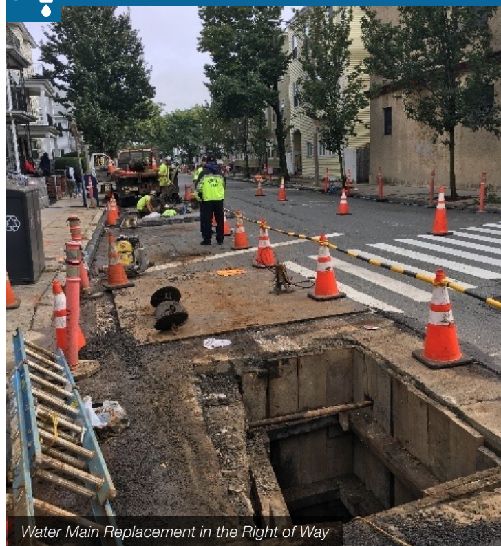
Water Service Lateral Replacement
